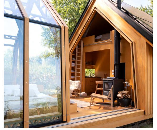
←↓ The cabin includes three "shells." Two of which slide along tracks: one glass and two wood and steel. The "shells" can overlap or open completely, permitting a variety of configurations with varying privacy. → The design stands out for its exposed wooden trusses, which provide strong structural integrity and lend the cabin its artisanal, crafted look.
