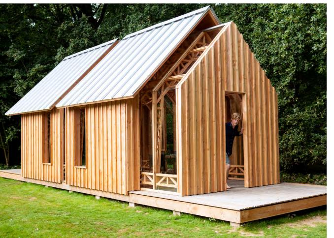
←↓ The mobile sections slide on industrial wheels along inbuilt tracks and can be rearranged simply by pulling them into the desired location. → Cabin Anna is primarily made of sustainable Accoya wood. Because it is relatively light, it can be installed in most places using only a screw foundation.
